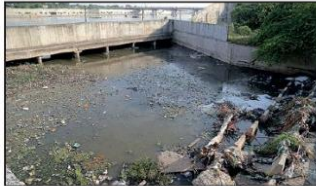
Chandrabhaga sewage outlet on riverfront near Sabarmati Ashram
